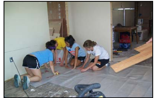
Students from the Academy of the Holy Angels installing new flooring.
